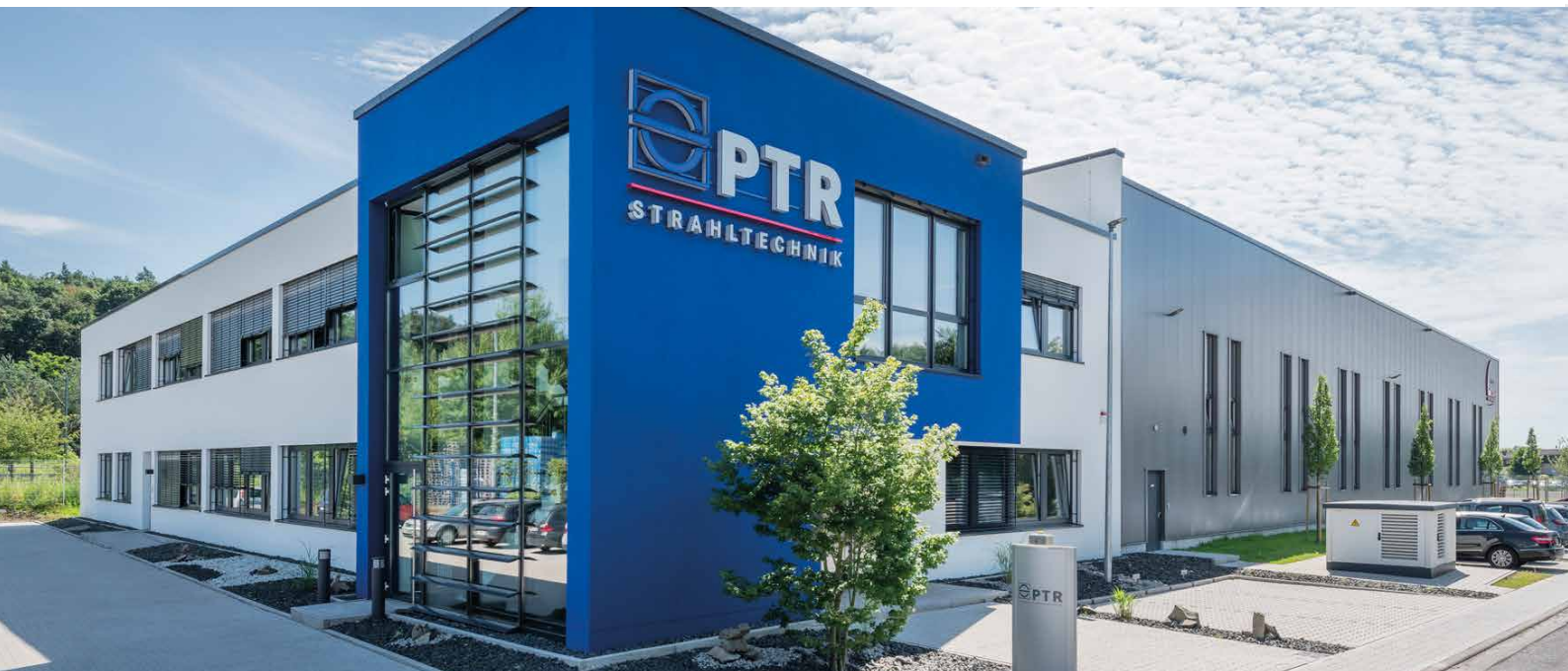
Location in Langenselbold (Frankfurt area)
